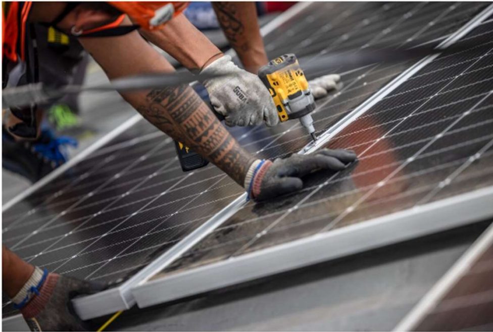
Workers install a solar panel in Barcelona. Photographer: Angel Garcia/Bloomberg
